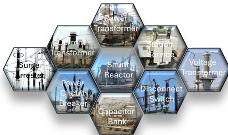
Figure 9.1: High Voltage Equipment Components
